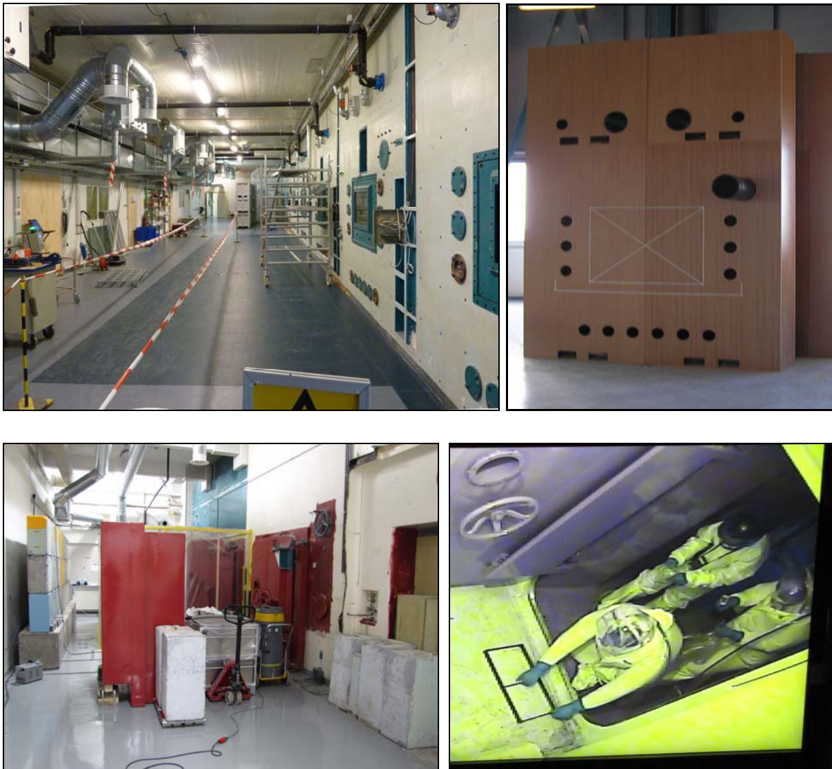
Figure 6. (top left) The operating hall with the front of the six concrete cells and newly installed ventilation systems; (top right) Full scale mock-up of Hot Cell no. 6 used for training of hotspot removal and first entry. (bottom left) tent and airtight seal-door access to a single cell used during the 2011 entrance (bottom right).
