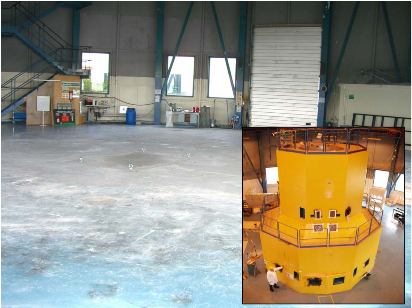
Figure 2. Cleaned up DR 2 reactor hall and floor with a removable concrete lid where the reactor once protruded the deck to the basement. Inset shows DR 2 reactor after removal of peripheral units.
